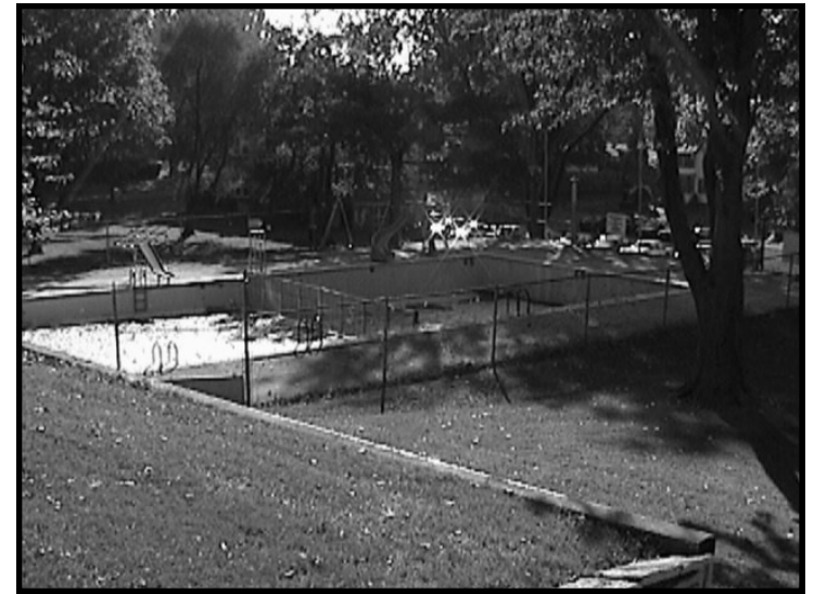
Construction of Cadzow Pool
